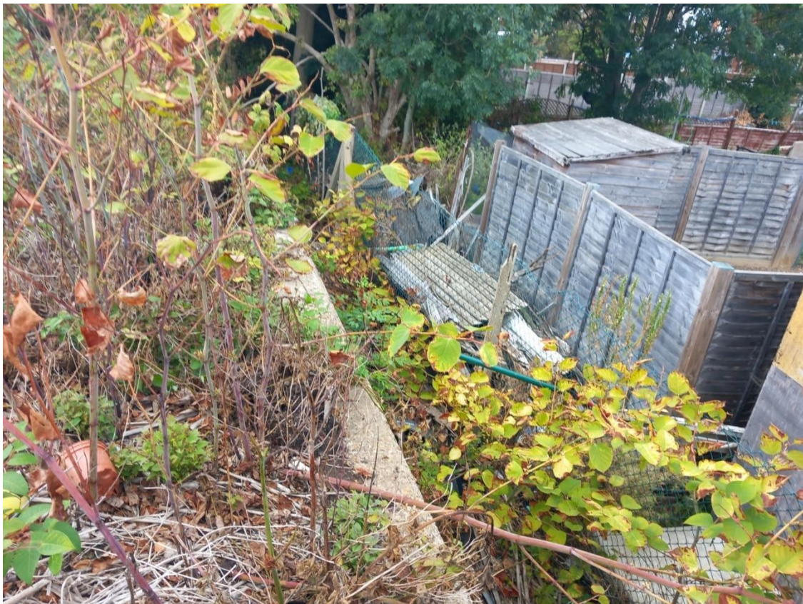
Boundary buffer and ground level changes from site to Pinner Road properties
