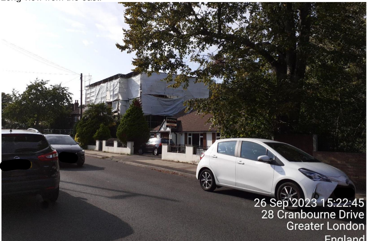
Long view from the east:
