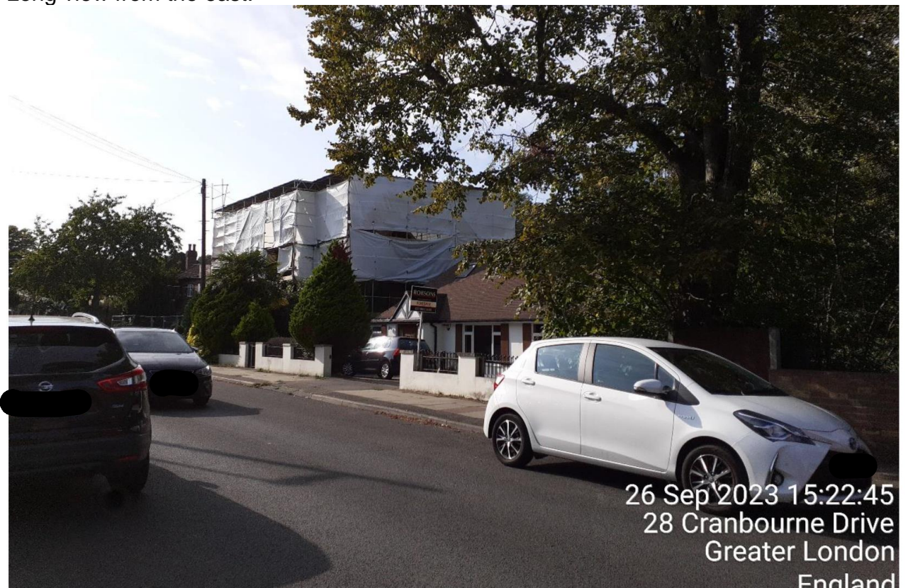
Long view from the east:
